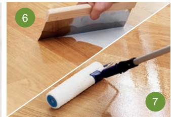
6 Apply finish with a trowel, then apply final finish using a roller
