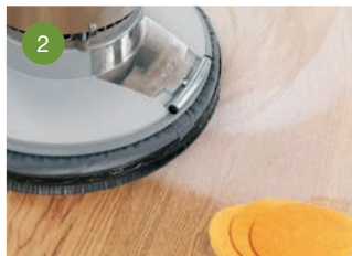
2 Superficial abrasion using Bona Diamond Abrasives (grit 80)
